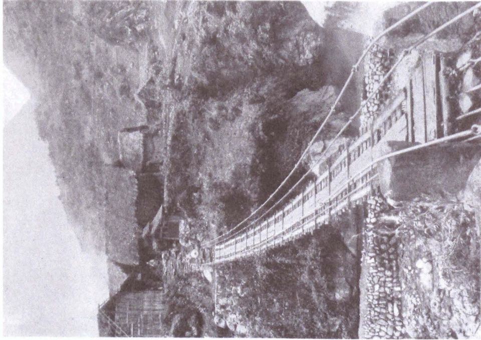
Primitive Suspension Bridge Skillfully Wrought by Workers in Iron and Steel With Crude Yet Effective Tools and Primitive Smelting Apparatus, Along the Chino-Tibetan Frontier
